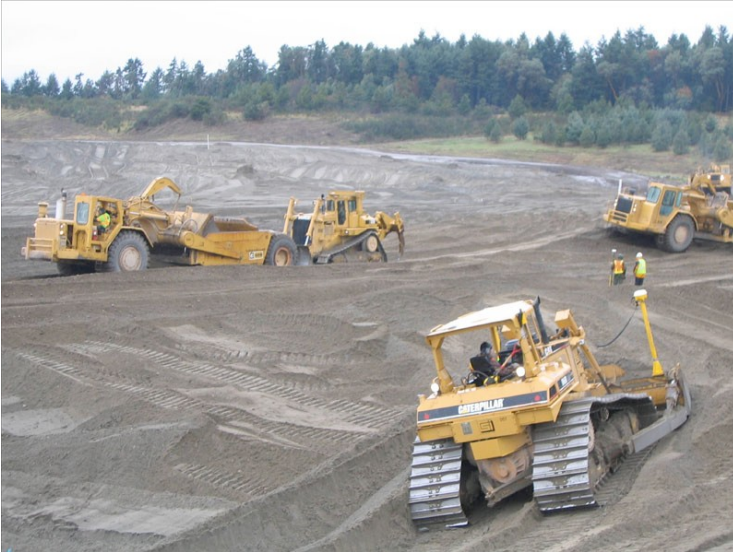
Mass Excavation Equipment at Work
