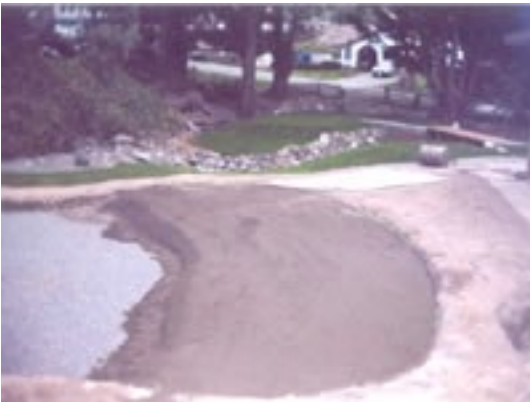
Greensmix being spread over gravel layer
