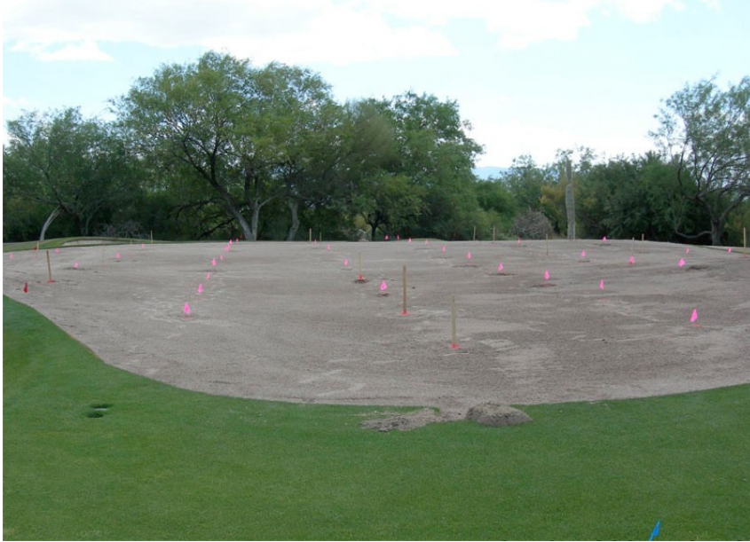
Putting Surface Under Construction
