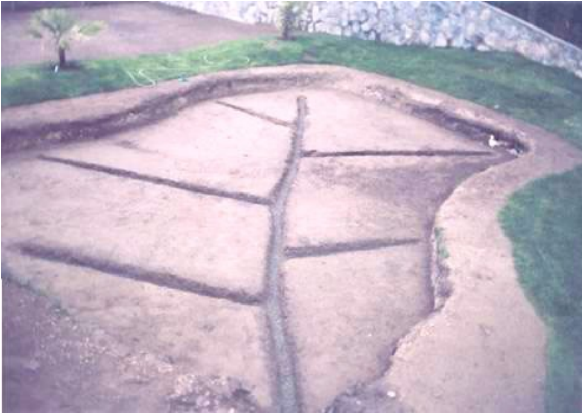
Trenches for perforated Pipe
